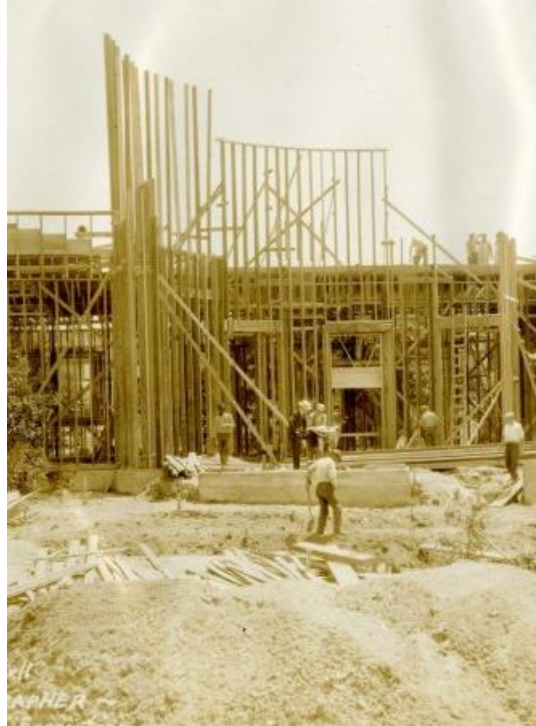
Illinois State Building under construction
